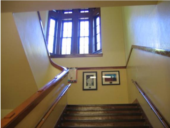
Staircase and handrail
